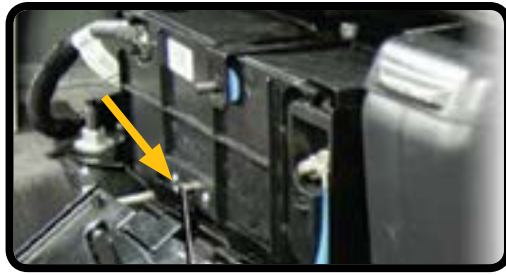
Disconnect Switch (shown with cover open)
