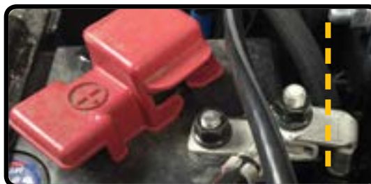
Cut the Positive Battery Cable
