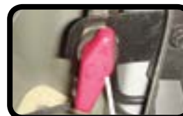
Manual Shutoff Valve
