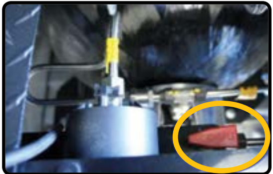
Turn Isolation Valve Counter Clockwise
