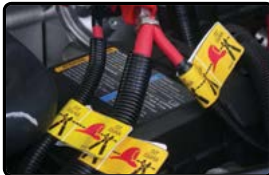
Cut 3 Exposed Cables (Alternate Procedure)
