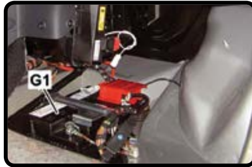
12V Battery Location
