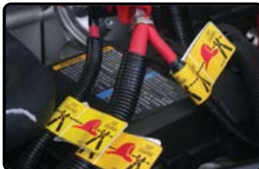
Cut 3 Exposed Cables (Alternate Procedure)
