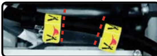
Cut 12V Battery Positive Cable As Marked
