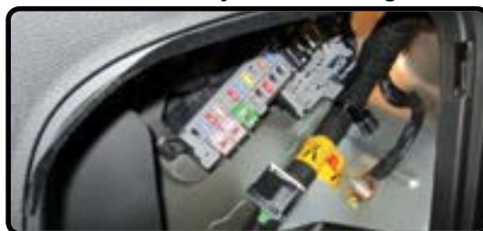
Cut 12V Positive Battery Cable
