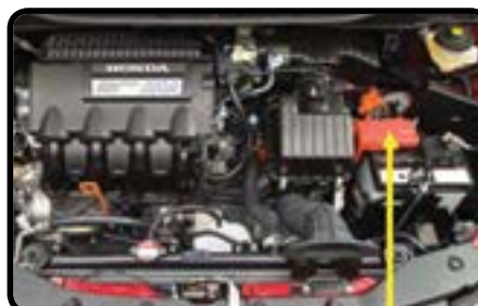
Positive Battery Terminal
