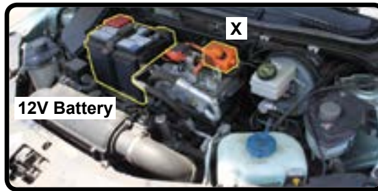
Battery and Service Interruption Location
