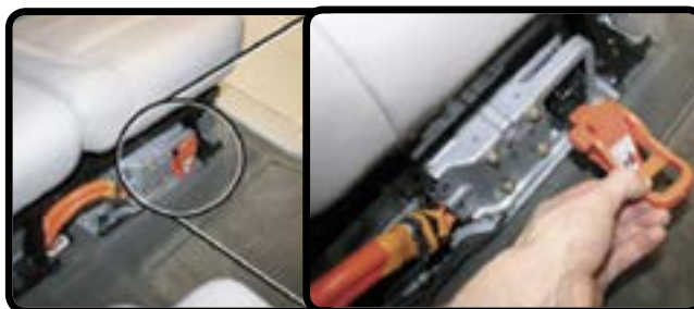
HV System Disconnect
