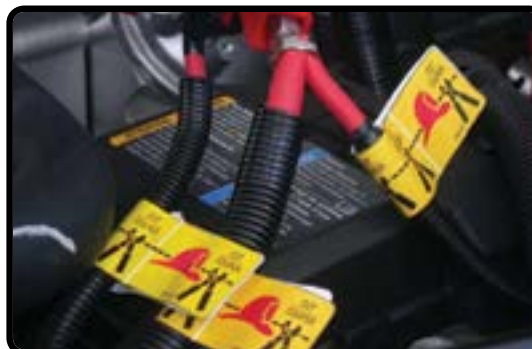
Cut 3 Exposed Cables (Alternate Procedure)
