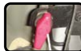
Manual Shutoff Valve
